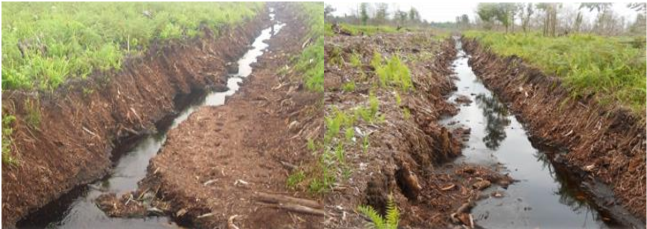
Figure 2. Large canals developed on peatland lowered water table level till the depth of the canals and dried up surface peat material
